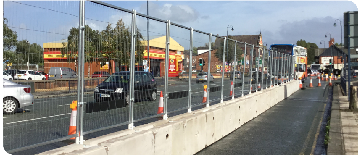
TVCB's with fence securing highway
